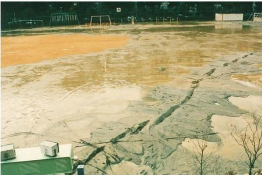
Artificial islands constructed by filling up soils were liquefied like this.
