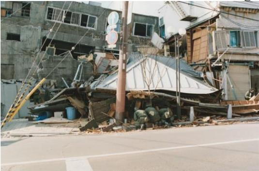
Houses were broken and the first floor was crushed and it seemed as if the second floor were the first floor.
